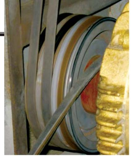
**An ongoing equipment-specific maintenance program can help prevent issues, such as a loose belt that has slipped off of a worn drive pulley, from becoming dilemmas.**
